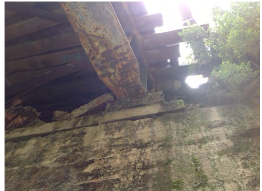
right bank upstream girder narrows at bearing
