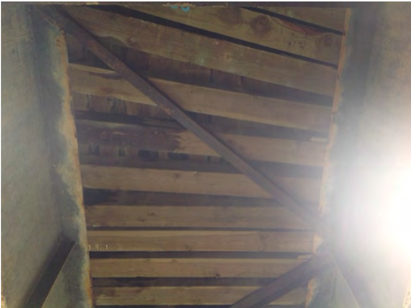
cross tie angle at right bank abutment
