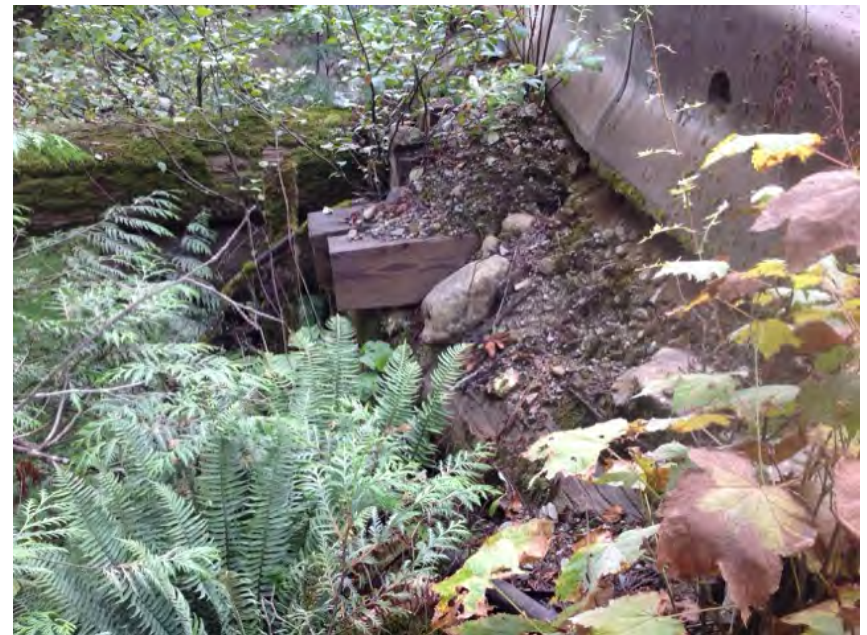
left downstream bank - ties and tiebacks retaining fill
