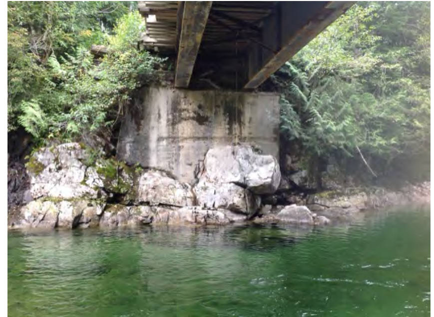
Left Bank Abutment when facing downstream
