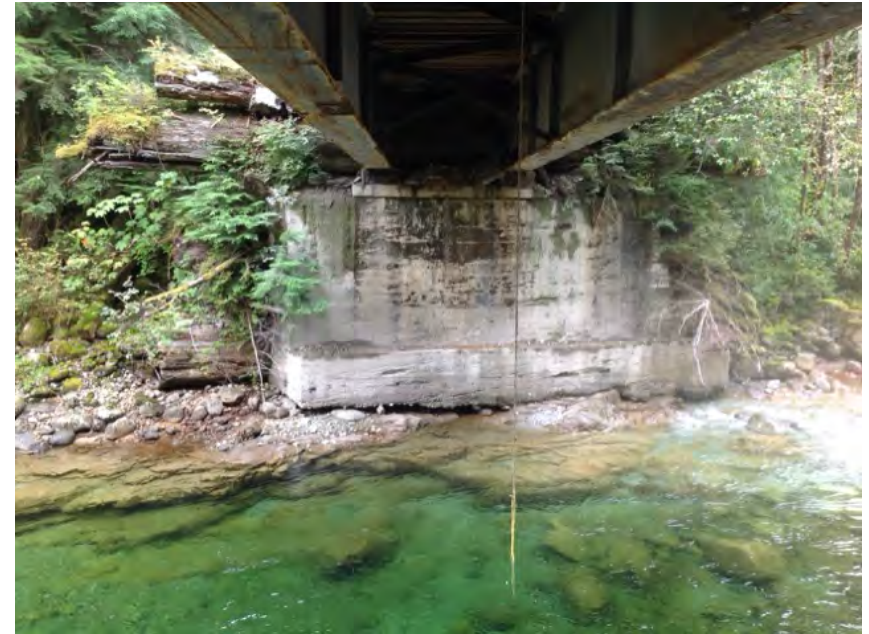
Right Bank Abutment when facing downstream
